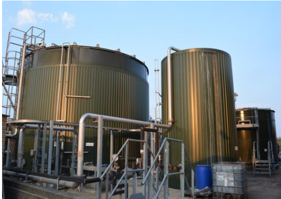
Technical scale demonstration of Se and Co supplementation to control digester stability
