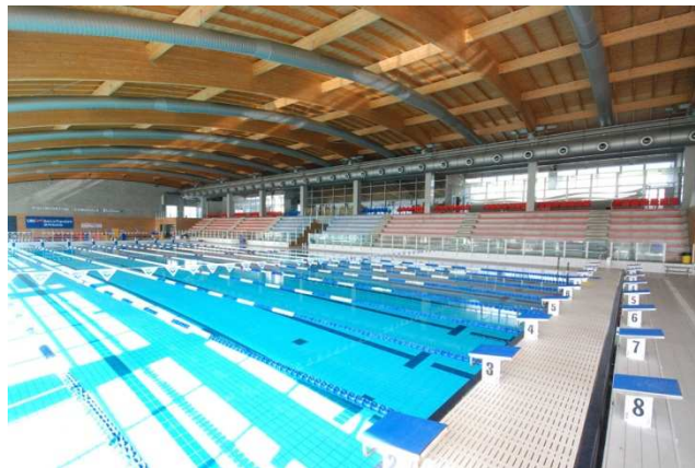
Swimming pools heating
