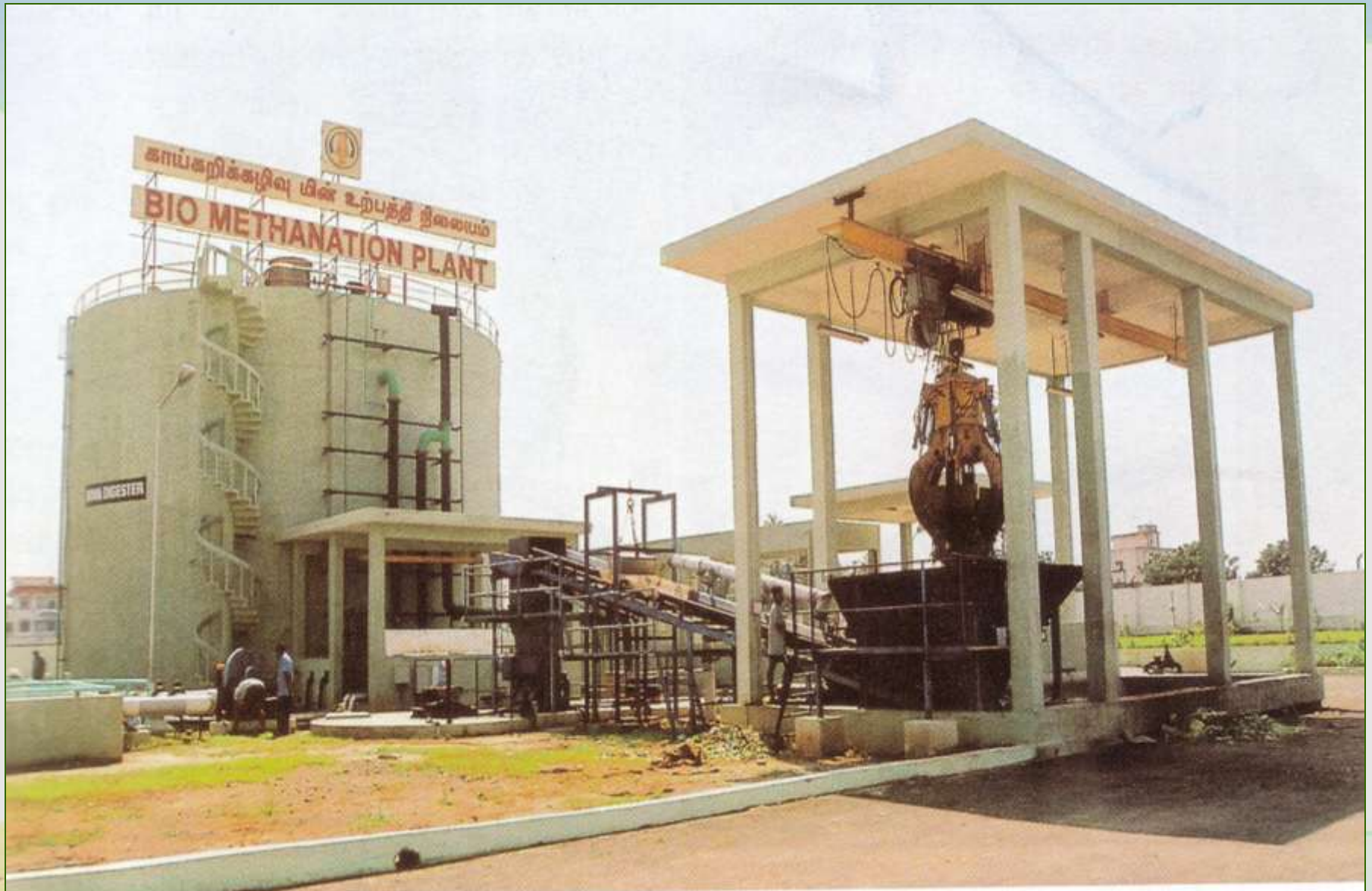
A 30 Tonne/ day capacity Vegetable Market based Biogas Plant at Chennai
