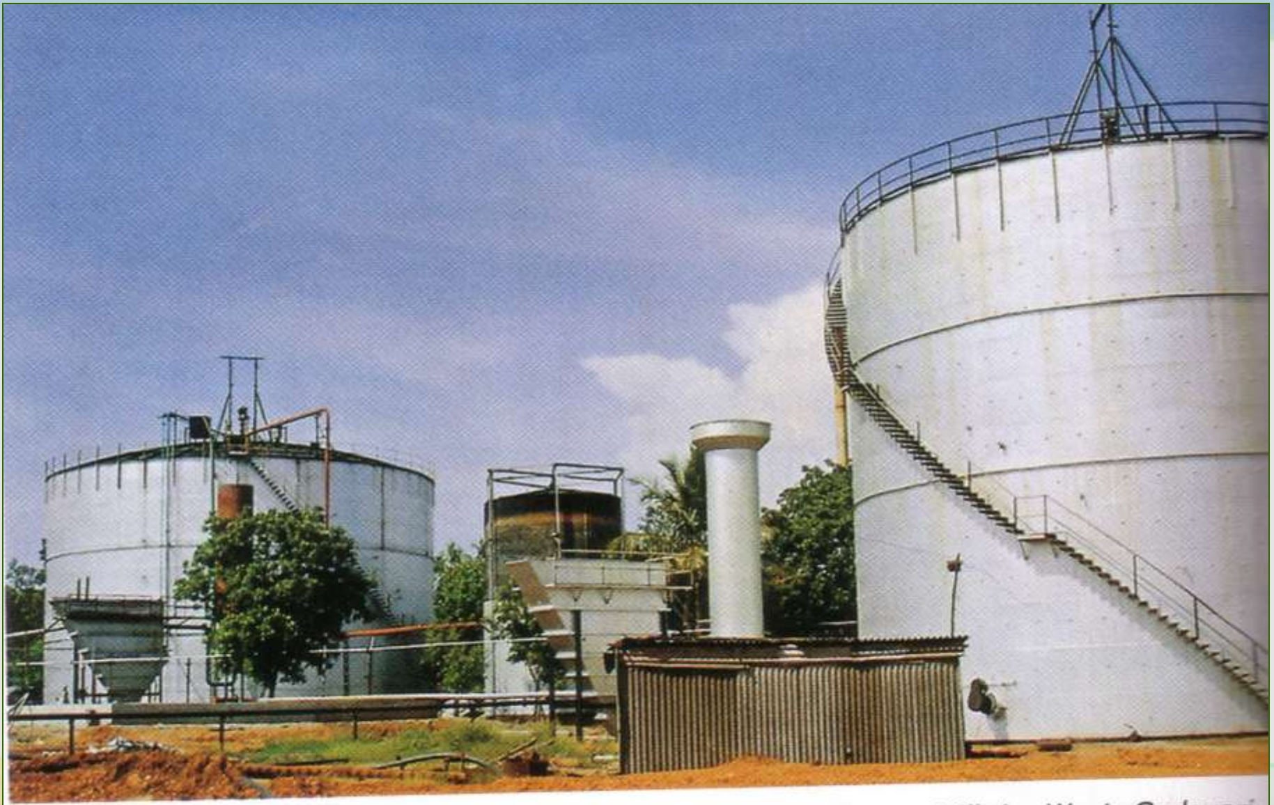
A 1 MW Distillery Effluent based Biogas Plant at a Sugar Mill in West Godavari Andhra Pradesh
