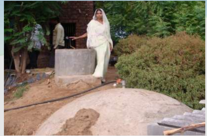
Deenbandhu 2m 3 model Family size biogas plant
