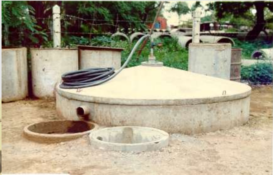
A Pre-fabricated RCC based Krishna model fixed dome Biogas Plant
