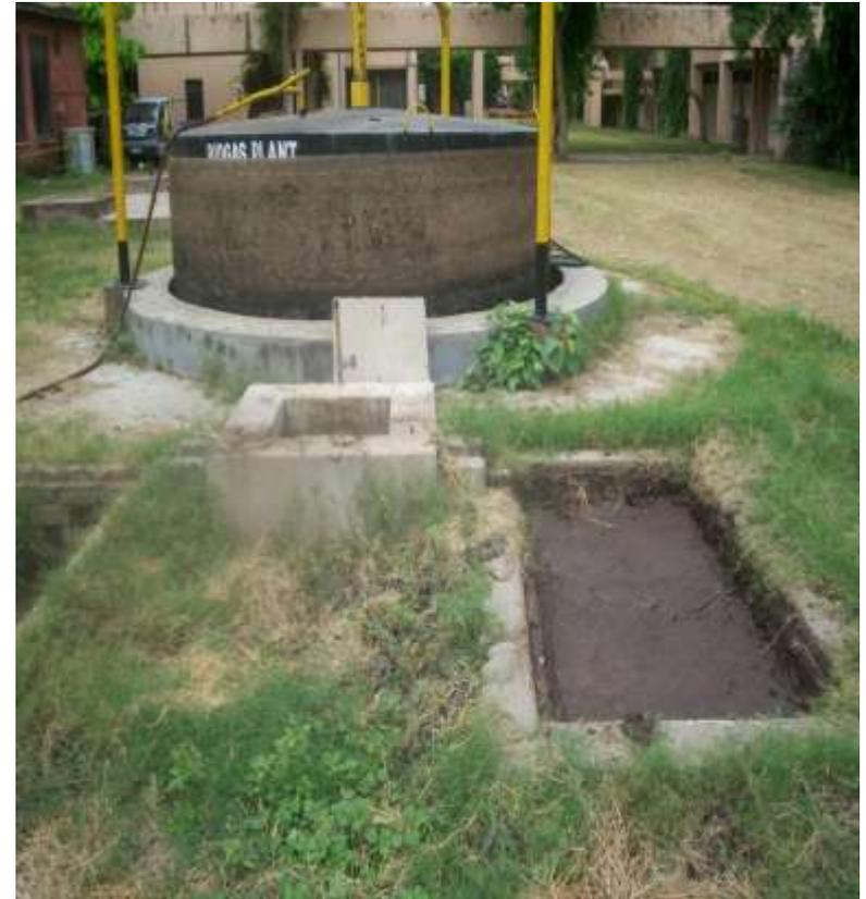
**Biogas plant (20 m<sup>3</sup>/d) being fed with jatropha & pongamia oil seed cakes**
