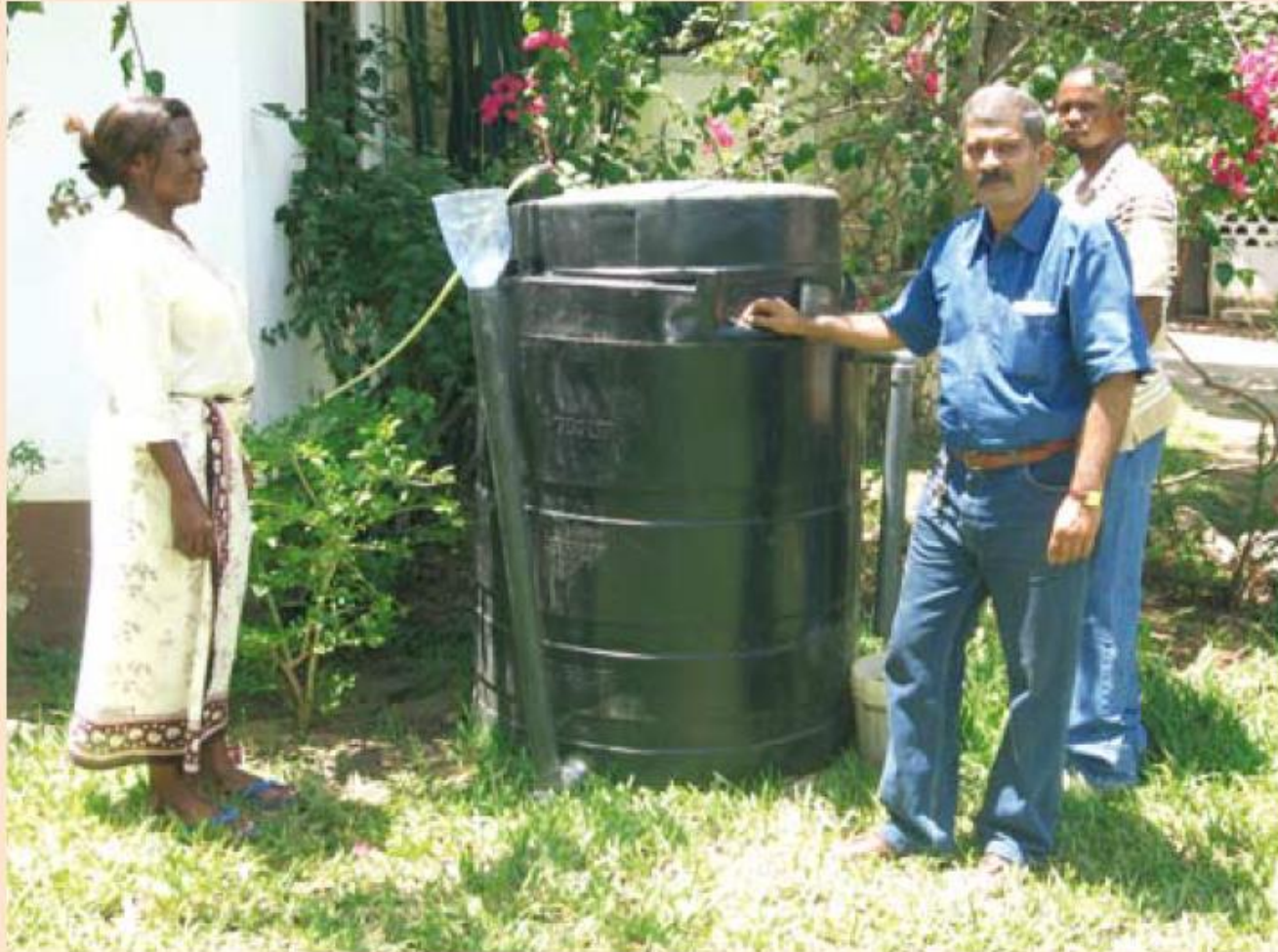
Photo 2: ARTI biogas plant in Dar es Salaam, Tanzania.
