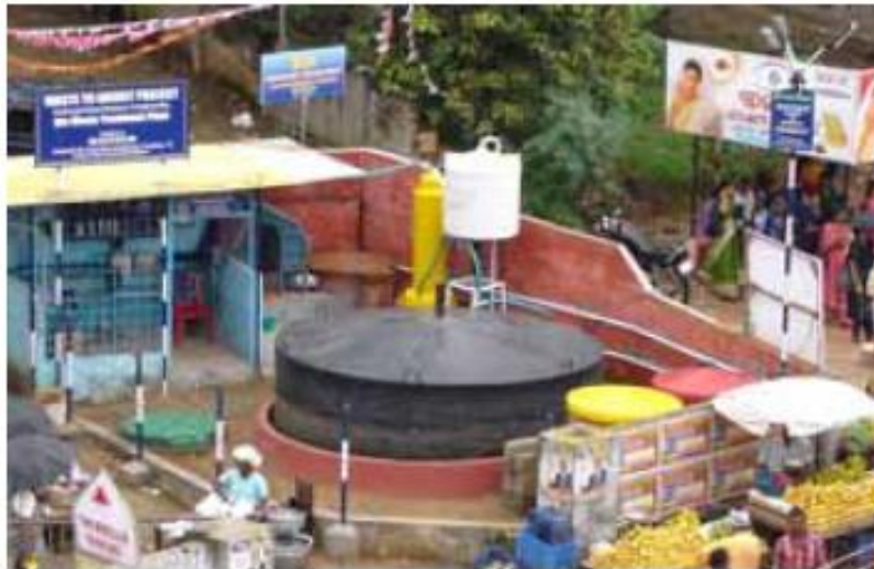
Picture 19: A BIOTECH plant treating organic solid waste on an institutional level.
