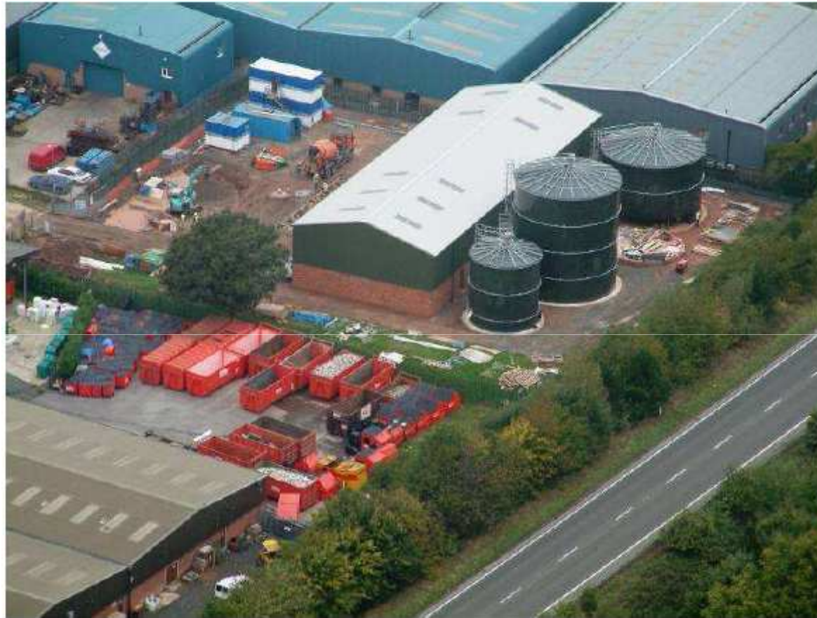
Ludlow biodigester under construction
