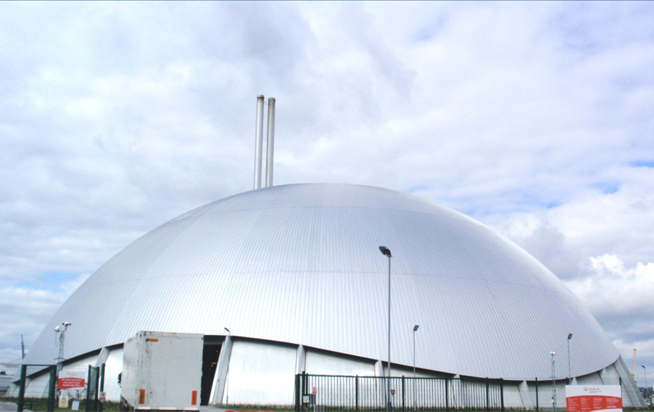
Energy Recovery Facility at Marchwood (Incineration) ©Anuda Tawatsin
