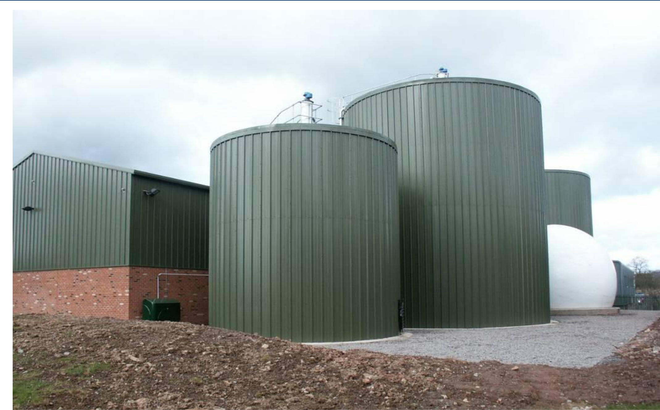
Anaerobic Digestion Plant at Ludlow ©BiogenGreenfinch
